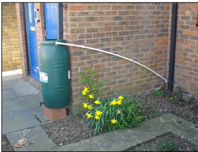
Figure 4-5 Example of a 100L water butt retrofitted to existing development
