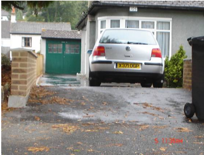
Figure 4-6 Raised Driveway, Croydon
