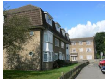
Bray Court to Sopwith Ave
