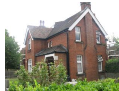
80 Coombe Road (built 1908)
