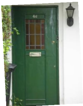
Original front door
