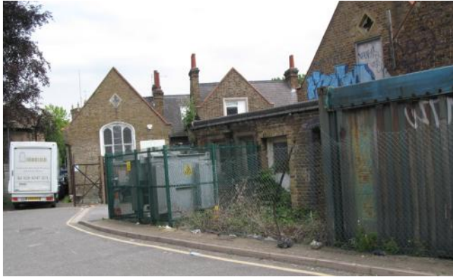
Victorian school, now with sub-station and extension, off Hawks Road
