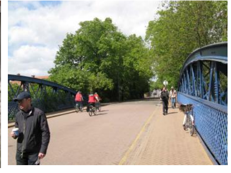
The Blue Bridge, Springfield Road
