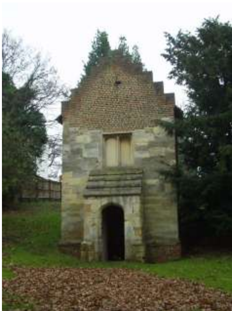
Coombe Conduit, lower house
