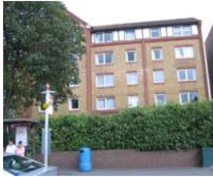
The flatblocks along Galsworthy Road
