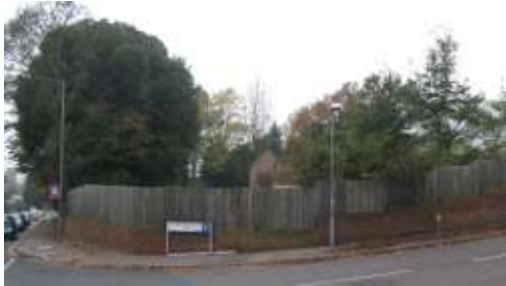
Coombe Conduit, obscured by fence
