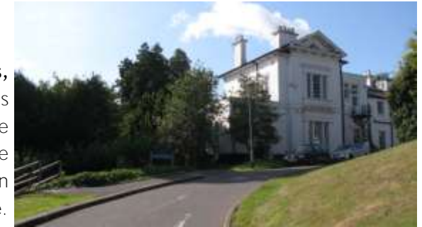
Coombe Hurst Building
