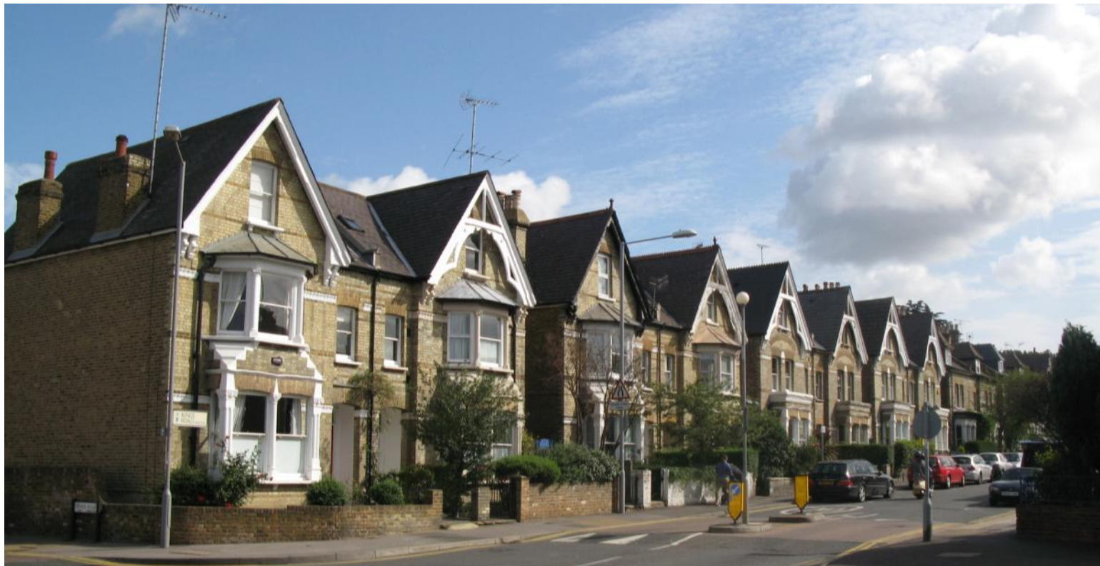
King's Road semi-detached 3-storey house type
