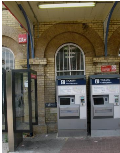
Daylight and architectural detailing need— lessly obscured by ticket machines
