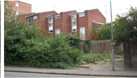
Kingston Hill could be improved by a public real project which addressed car dominance and took advantage of the wasted edge spaces
