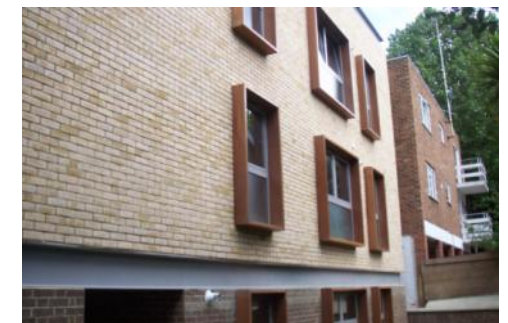
48 Kingston Hill let down by landscape character and parking inside the non-car entrance
