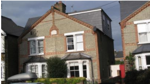
A degraded roofscape
