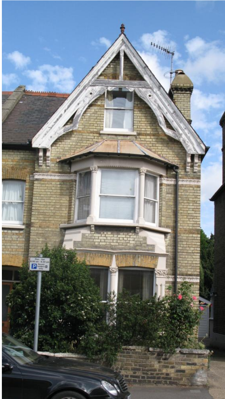
King's Road semi-detached house type with original features
