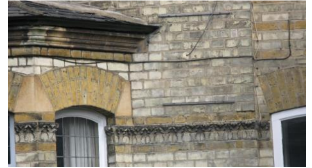
Victorian building line detail
