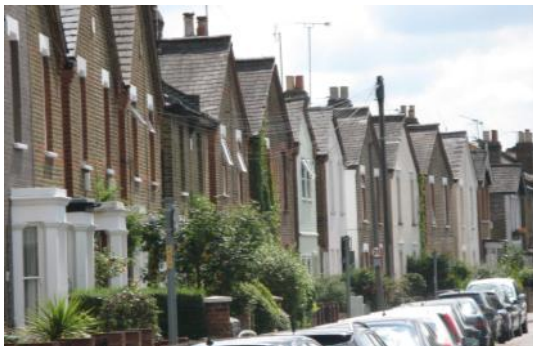
An intact roofscape
