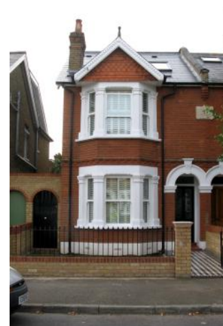
A refurbished house with new front boundary and garden gate
