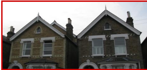
The more recent trend to roof enlargement by building a piggy-back roof
