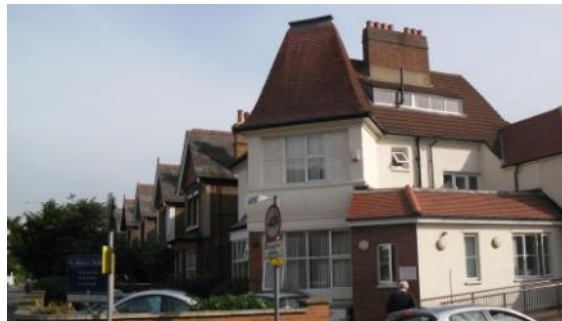
Built as a Victorian feature on a prominent corner, originally with a 'Gothic' mansard roof, now engrossed by enlargement, its modelling swamped, trees, subtle detailing and materials removed and the frontage has become a car-park
