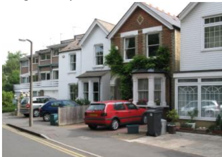
Front garden walls removed weakening
