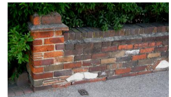
An original front boundary
