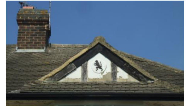
Typical gable above a 2-storey front bay
