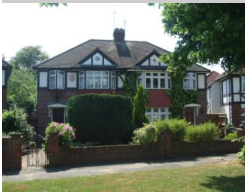
Semi-detached house type, note different arrangement of architectural elements
