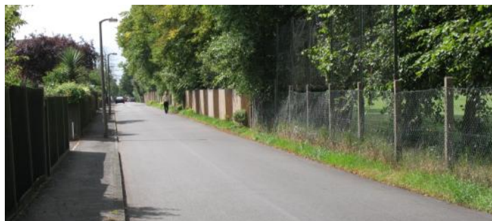
Lower Ham Road close to Richmond Road
