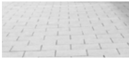
1. Option A Flag paver Pre-cast concrete granite aggregate flag pavers or setts
