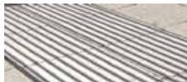
7. Hazard pavers Pre-cast concrete corduroy paver (contrast colour) for top and bottom of steps
