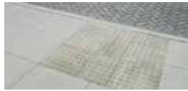
5. Tactile blister paver Pre-cast concrete blister paver (contrast colour) for carriageway crossing points
