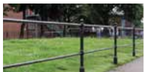
13. Railing Cast iron black post and rail
