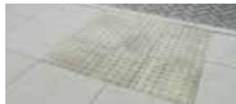
6. Tactile blister paver Pre-cast concrete blister paver (contrast colour) for carriageway crossing points
