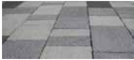
1. Option B SUDs Flag paver Permeable paver exposed aggregate textured pre-cast concrete paver
