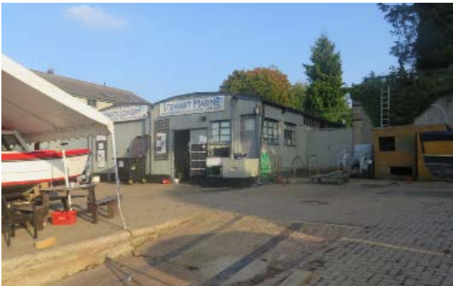
Fig 85 There is some industrial activity with a number of small businesses based at the boat yard at the southern end of Queens Promenade
