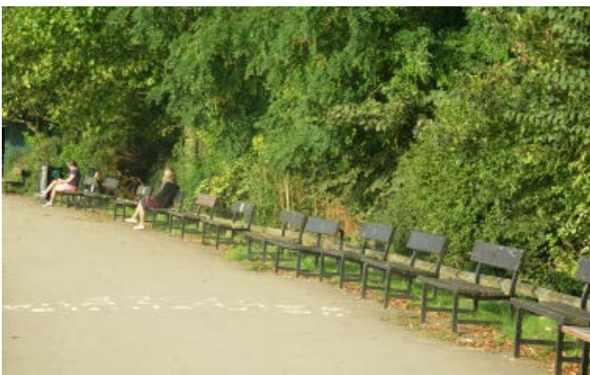
Fig 77 The Promenade is lined with memorial benches and the formal Victorian planting is now looking tired.
