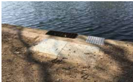
Retained concrete edges
