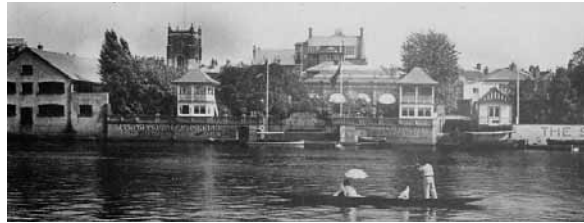
Figure 3.29: View looking east across the River Thames towards Nuthall's Restaurant garden.
