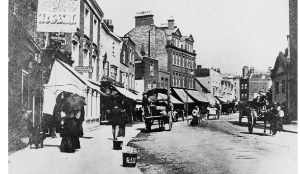
Figure 3.25: West side of the High Street c.1890
