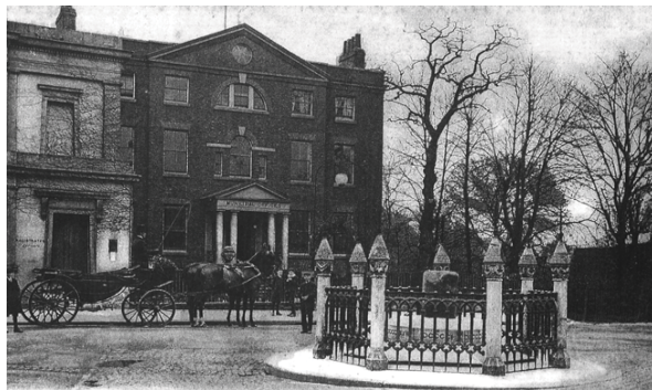
Figure 3.21: Coronation Stone and Clattern House c.1900
