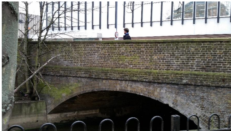
Figure 58 Hogsmill river bridge crossing
