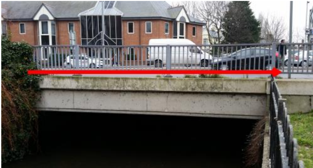
Figure 11 Hogsmill River crossing along Wheatfield Way
