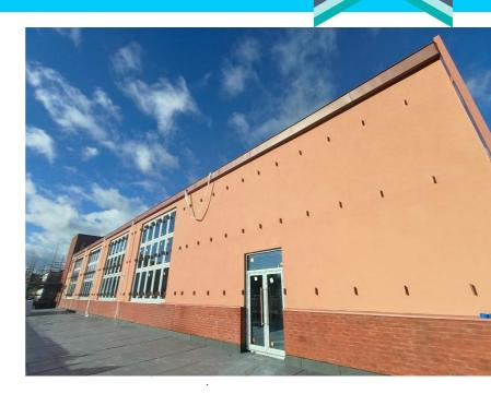
Externally, scaffolding is being dismantled to reveal the striking terracotta render, soon to be clad with panels to give the building its final layer. The pyramid roofs are complete topped with 'Monodraught' systems allowing the building to breathe naturally throughout the seasons.
