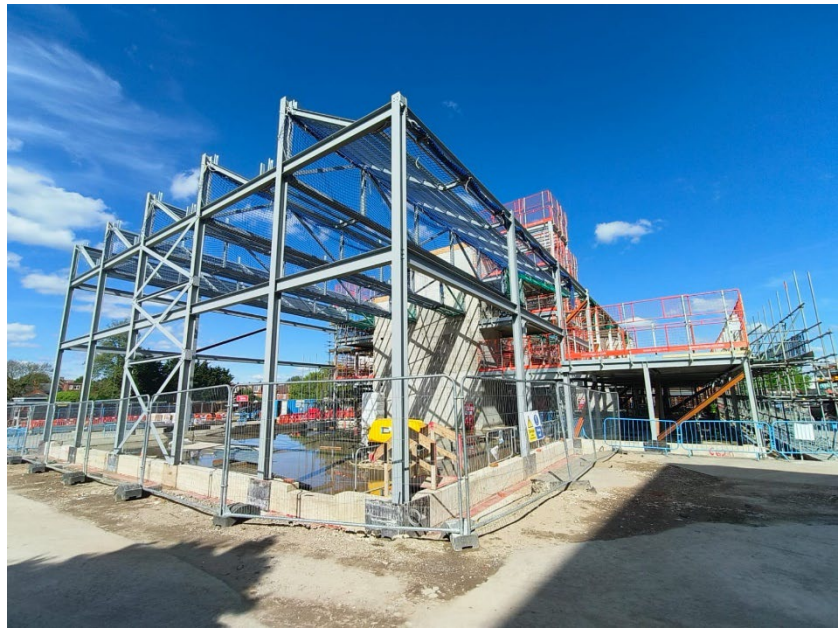
Sam Haile's shot of the completed steel frame in the April Sunshine
