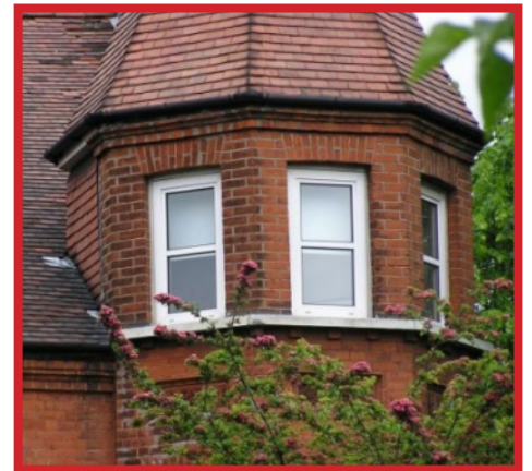
Building with uPVC windows
