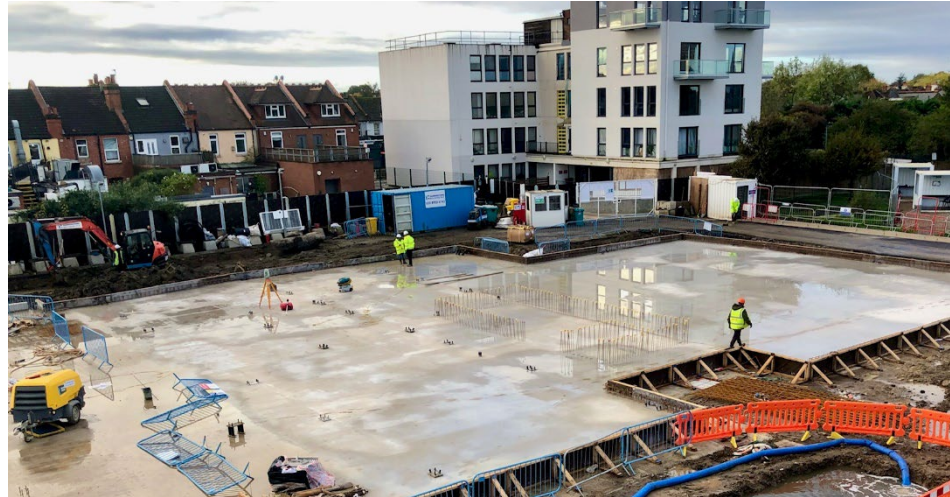
The ground floor slab is now complete
