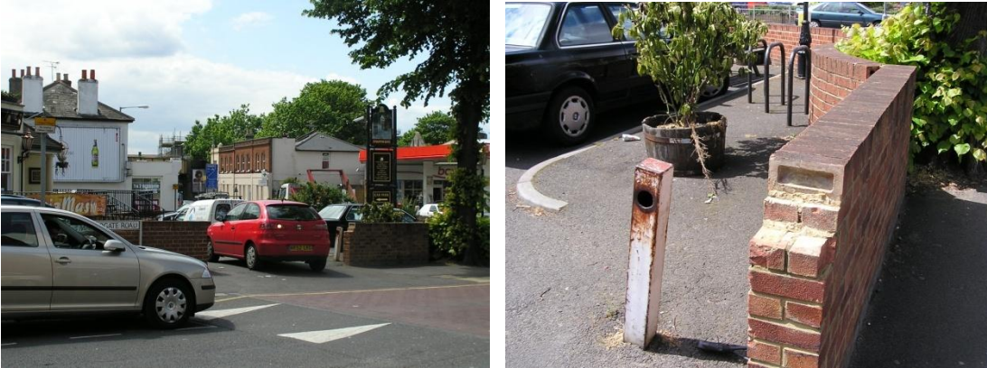
The Kingston Gate forecourt is unsightly, both in scale and in detail
