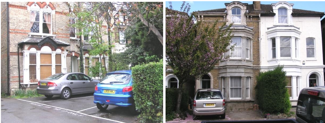
Damage: intrusive parking at 17 Kingston Hill; hard-standings at 2-12 Clifton Rd
