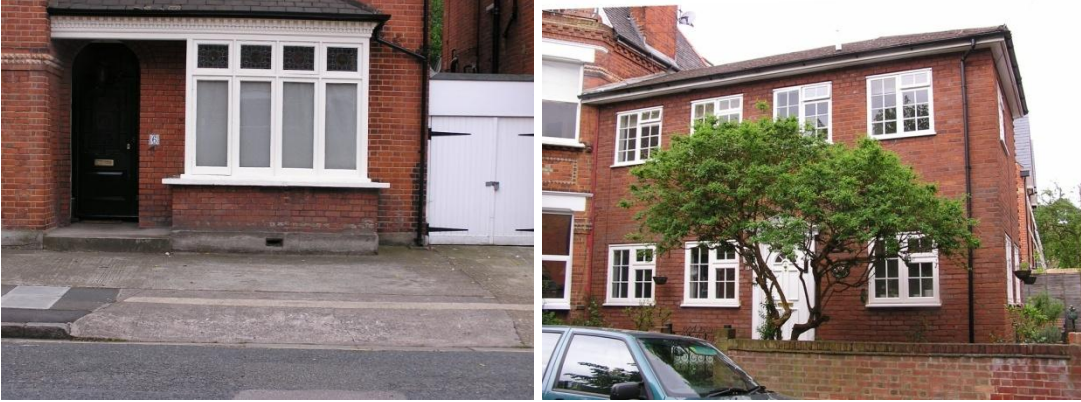
Hard-standings and unsympathetic extensions have affected the townscape quality
