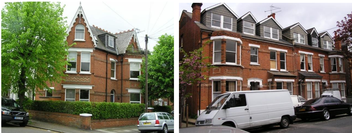
The corner gable in Brunswick Road is charming, but the dormer additions down the road are disastrous
