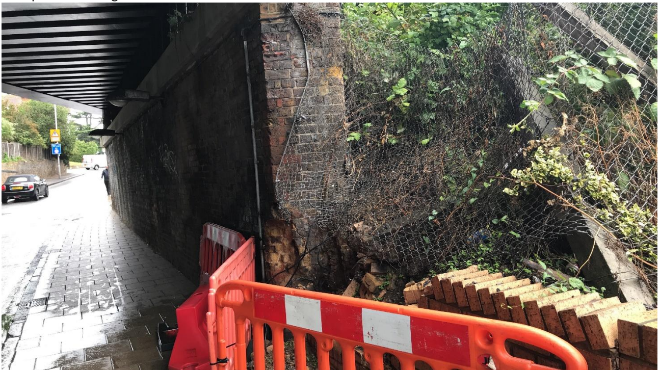
Collapsed retaining wall:
