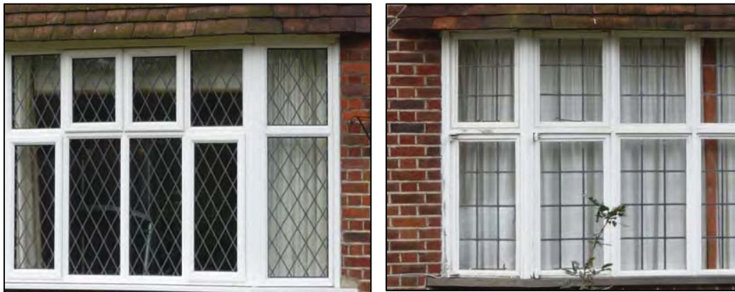
uPVC replacement windows. original wood and metal windows
