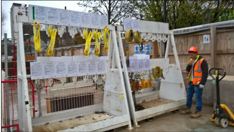
Figure 16 – Storage of Lifting Straps
