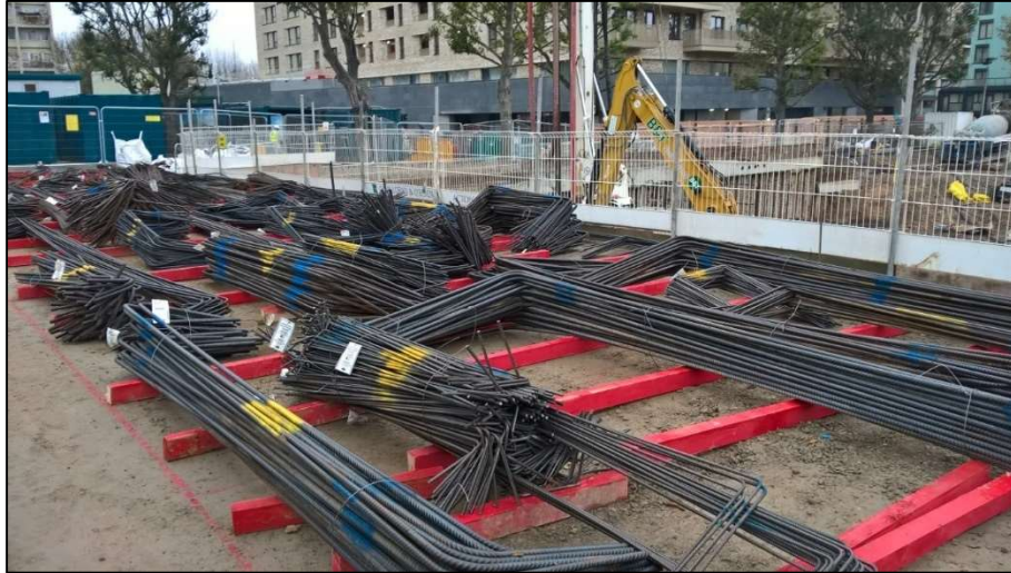
Figure 13 – Neat stacking of Steel Reinforcement
