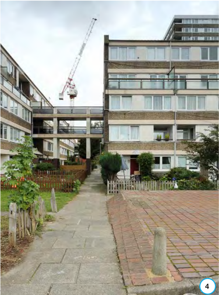
Figure 15: Shelford building - elevated passageway.
