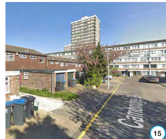
Figure 43: Fenced front gardens with mix of hard surfaces.
