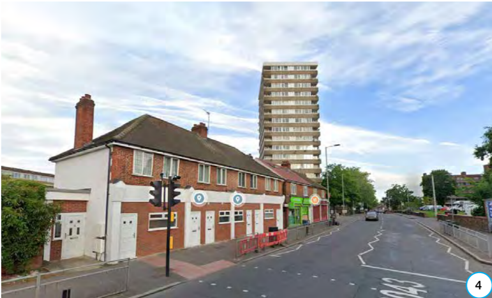
Figure 48: Cambridge Road - Local shops.
