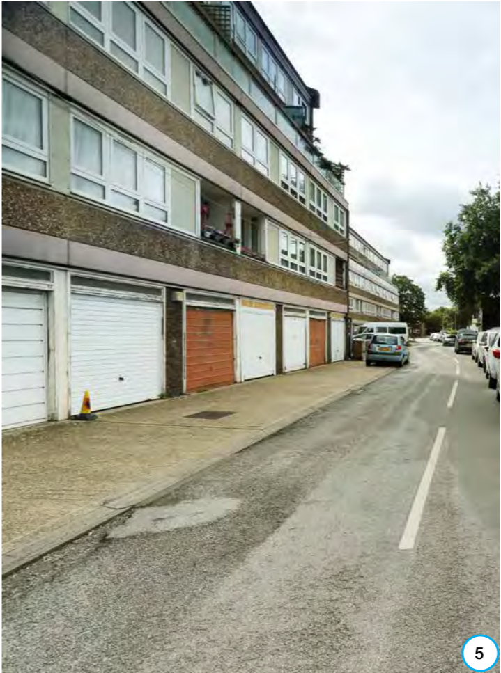
Figure 16: Comberton building - ground floor garages.
