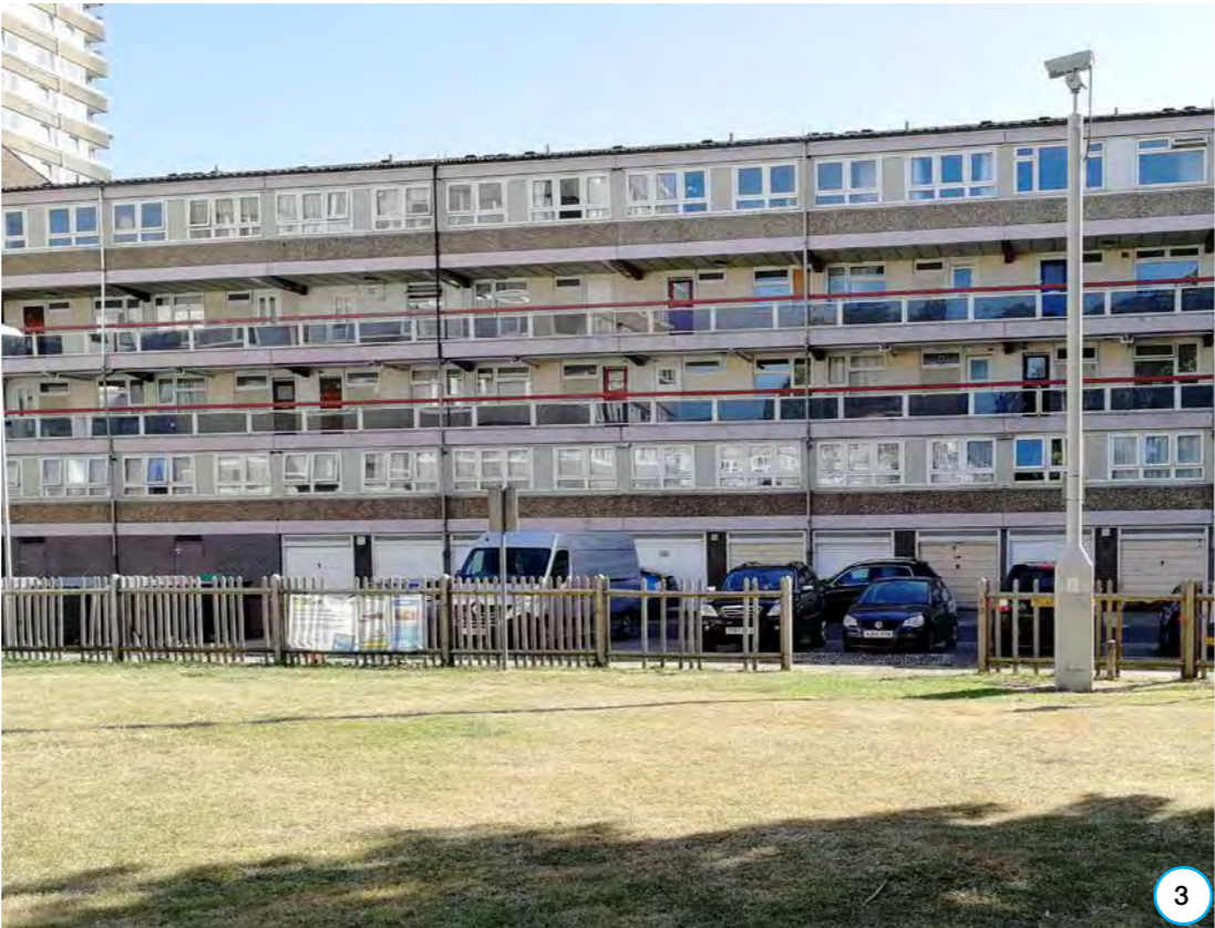
Figure 14: Westwick building - typical linear low-rise buildings.
