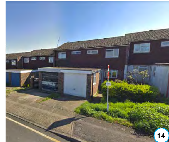
Figure 42: Fenced front gardens with mix of hard surfaces.
