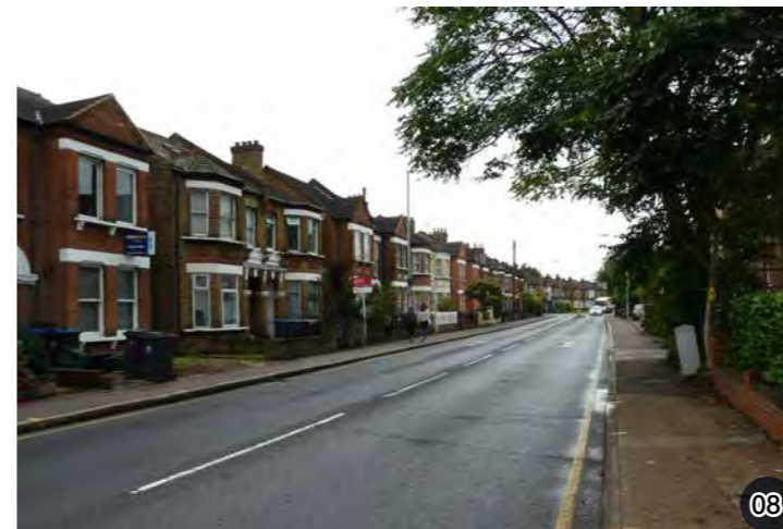
Figure 76: Hawks Road - street view.
