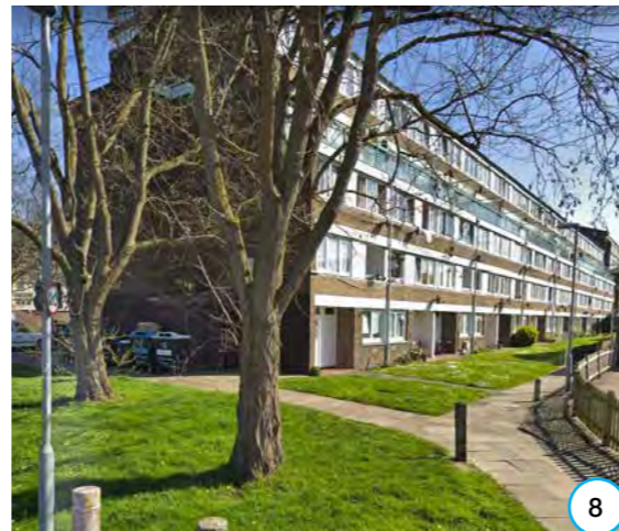
Figure 36: Green open spaces at ground. Refuse bins located within space.
