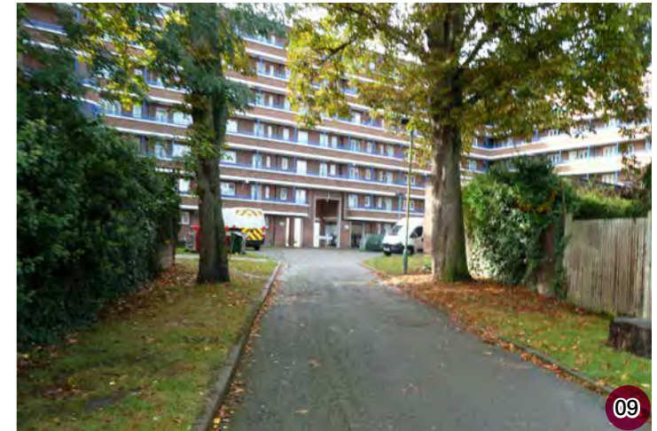
Figure 79: Cambridge Gardens Estate - street view.
