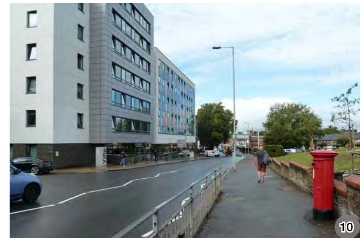
Figure 82: Cambridge Road - street view.
