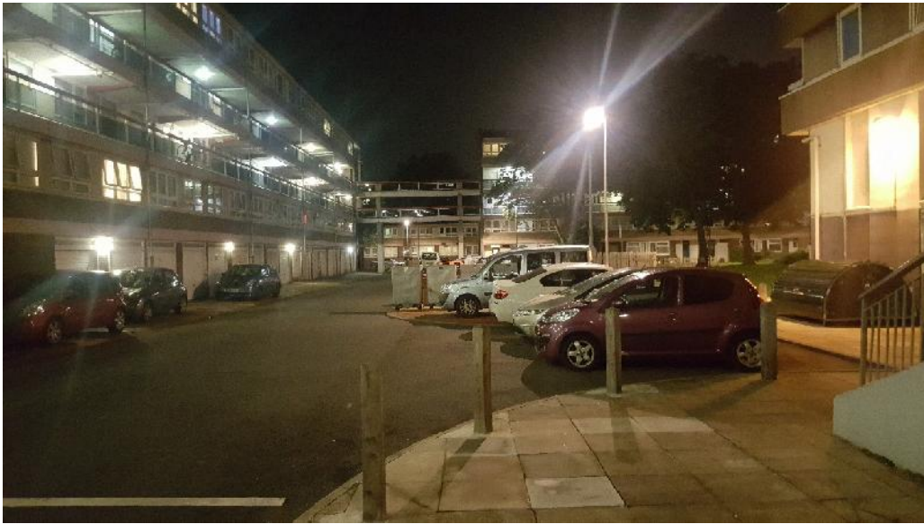
Figure 5.1 High levels of external lighting
