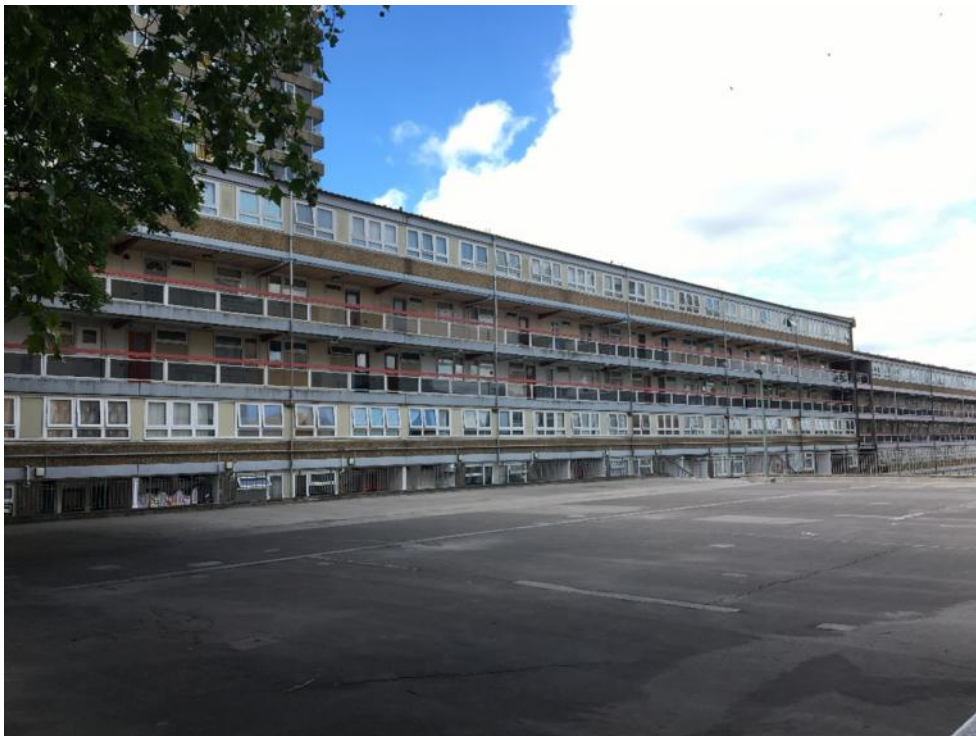
Figure 5.2 Unvegetated areas of hardstanding
