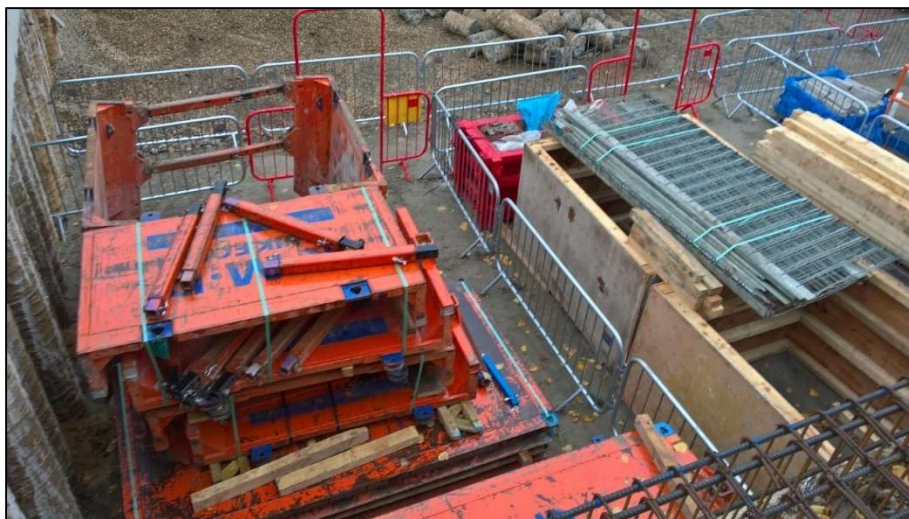
Figure 15 – Neat stacking of Formwork
