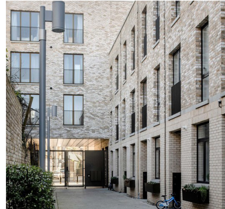
Figure 5.138: Off-street demised parking area to Townhouses.
