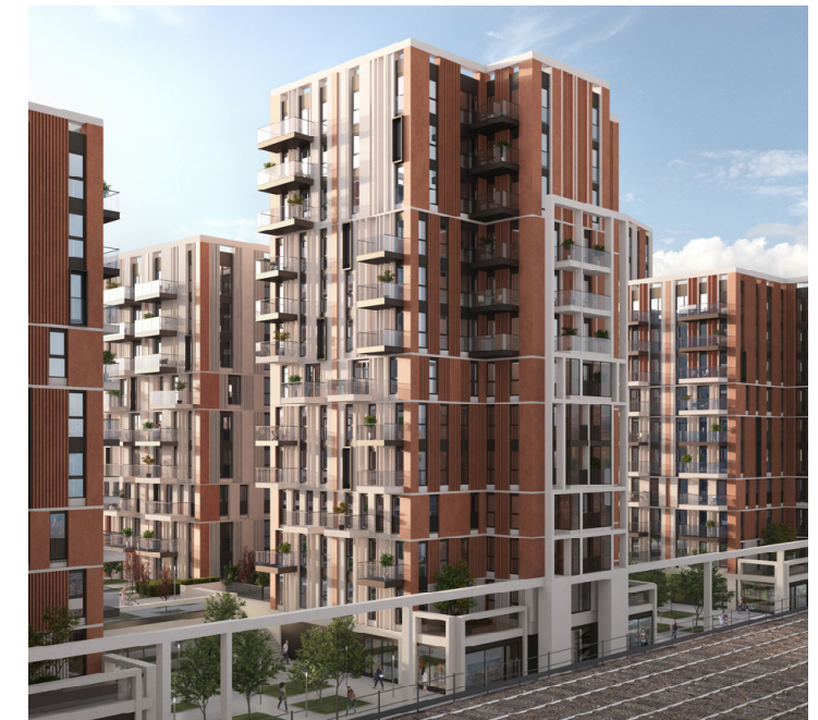
Figure 5.173: Exploiting dual aspect views from Mansion buildings Ponton Road - London - Patel Taylor.
