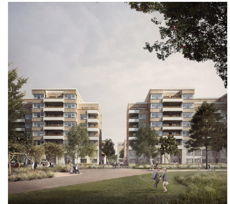
Figure 5.176: Gateway between two Mansion buildings. London - Mae Architects.
