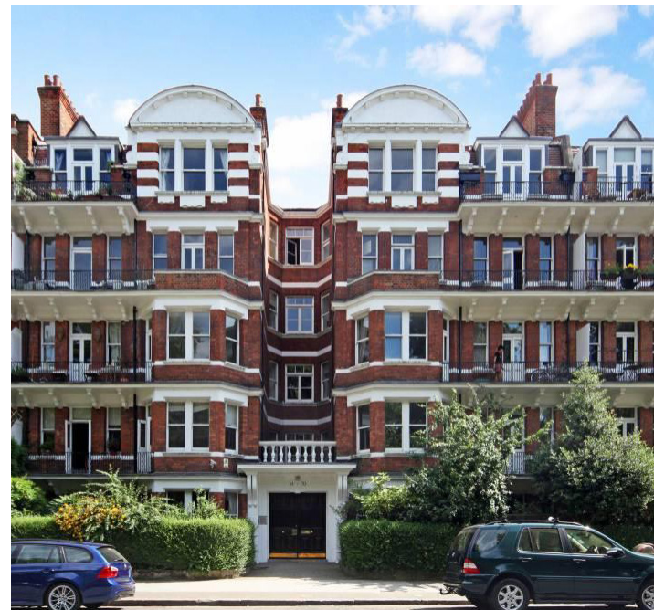
Figure 5.174: Traditional Mansion buildings with a shared communal entrance Prince of Wales Drive- London.
