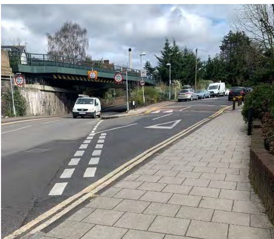
5. Coombe Road/Norbiton station approach
