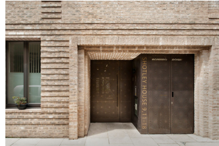
Figure 4.11: Entrances clearly expressed within base element.
