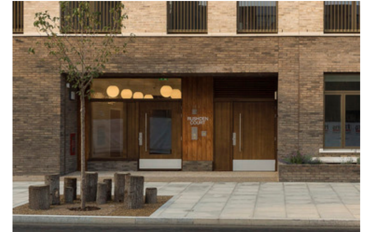
Figure 4.12: Entrances clearly expressed within base element.
