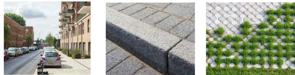
Parking Spaces - permeable concrete pavers
