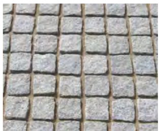
Amenity - concrete pavers
