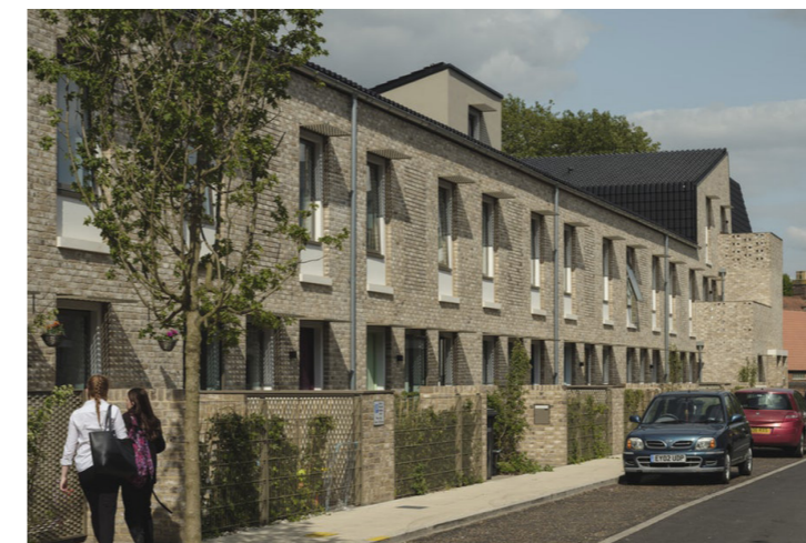
Figure 4.62: Low level brick wall interspersed with planting.
