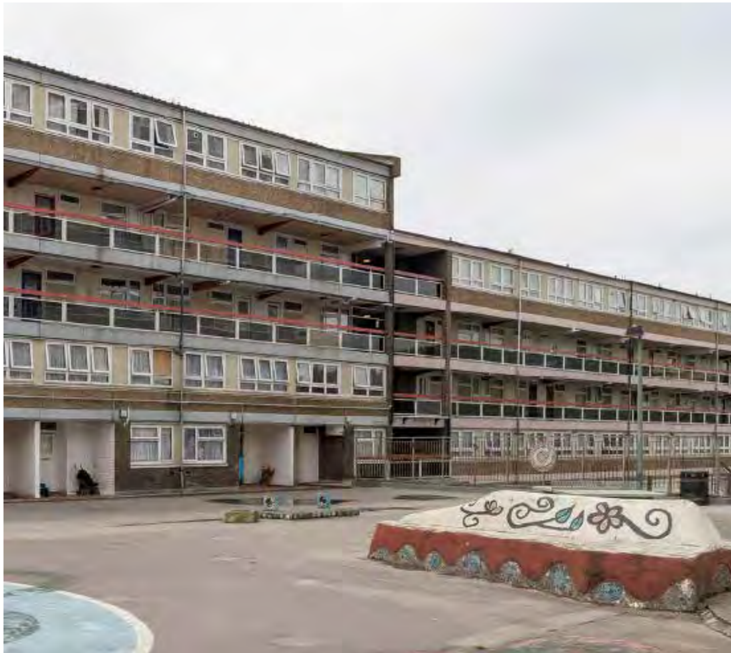
Figure 6: Carpark rooftop play space.
