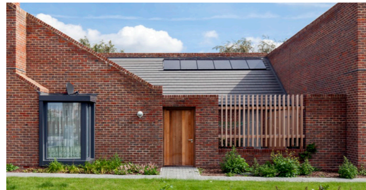
Figure 5.123: Precedent - Integrated garden walls, gates and screening Courtyard Housing - Barking - London - Patel Taylor
