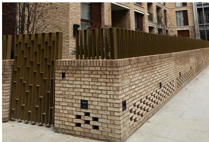
Figure 4.89: Low level brick wall with metal railing for privacy.
