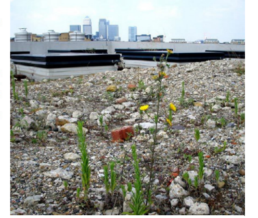
Figure 4.125: Precedent image of ballasted biodiverse roof.
