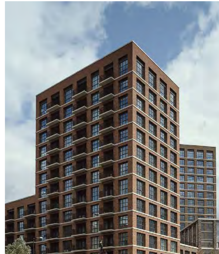
Figure 96: Macreanor Lavington, Porters Edge
