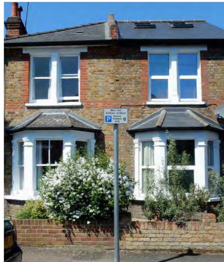
Figure 41: Example of a paired windows on Piper Road
