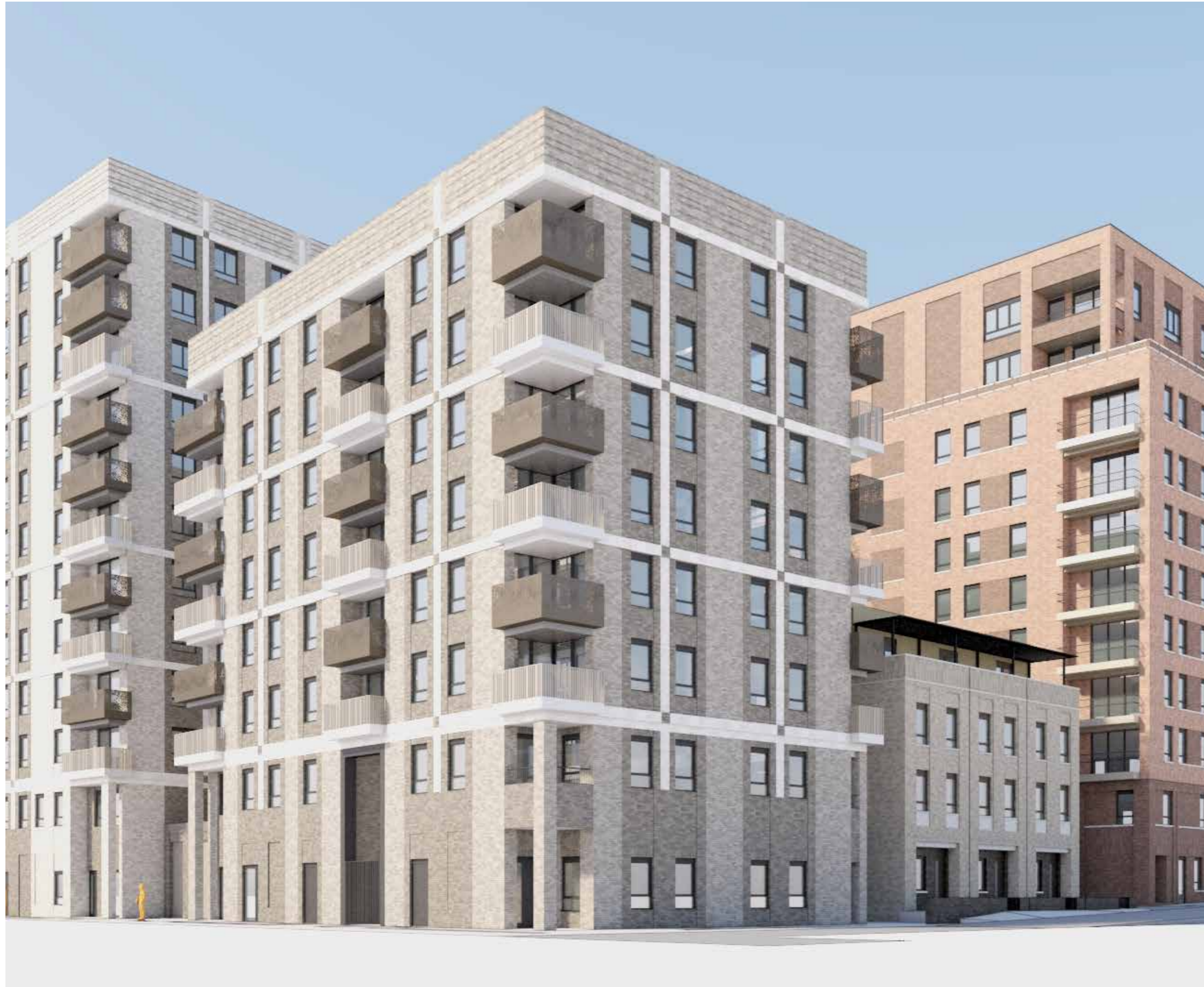
Figure 91: Render of Plot E. View looking north-east towards Buildings E4, E5 and E3
