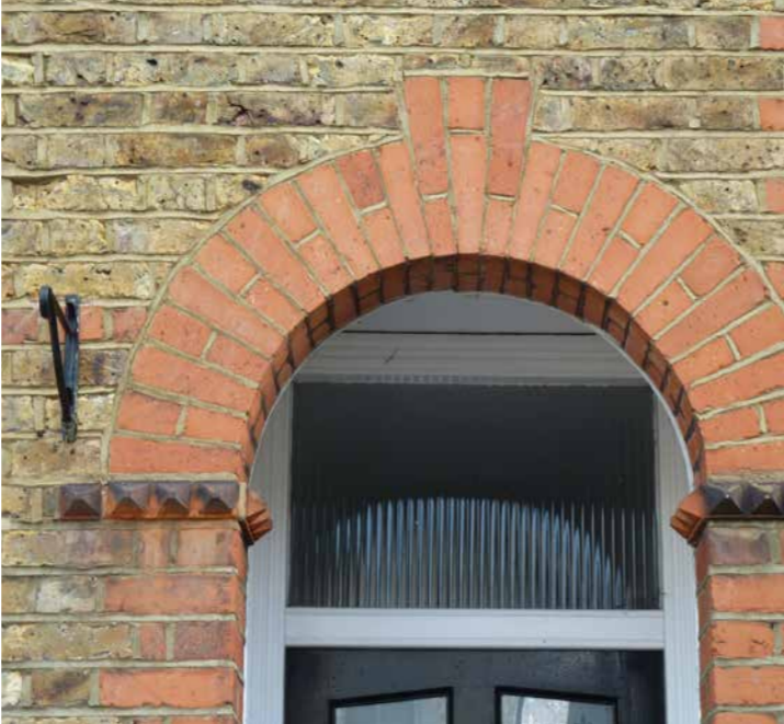
Figure 19: Example of door detailing on Chatham Road
