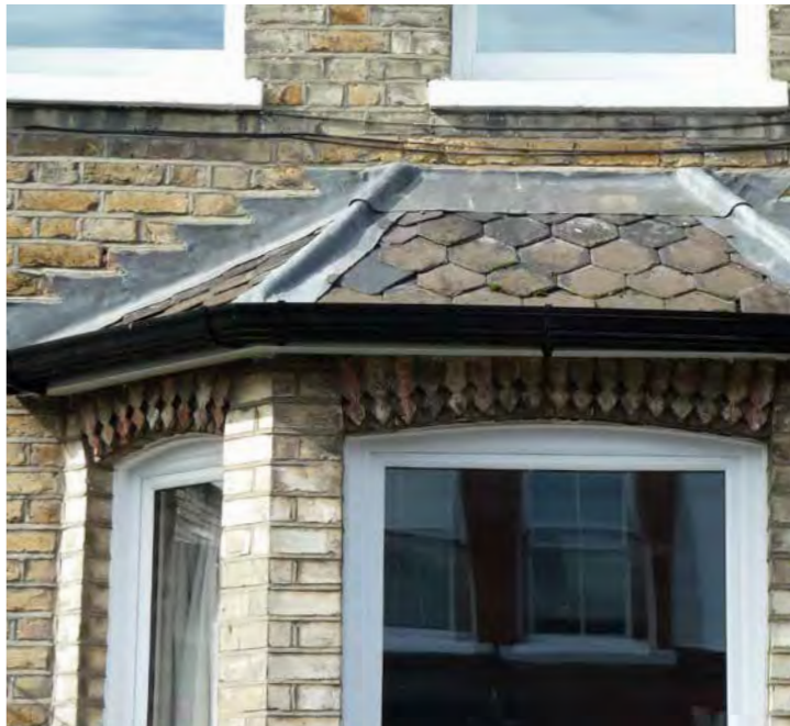
Figure 20: Example of bay window on Chatham Road
