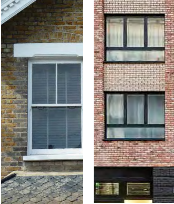
Figure 55: Window details on Chesham Road and Pitman Tozer's Monier Road November 2020
