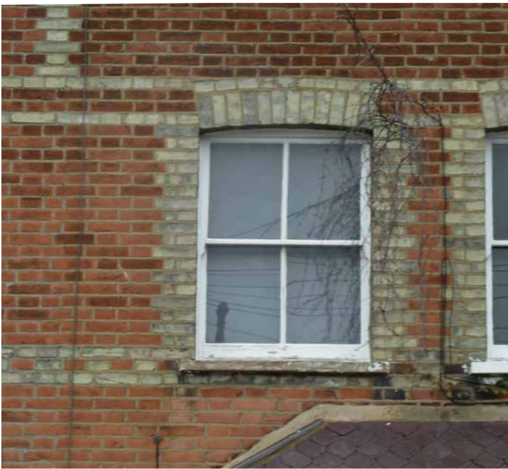
Figure 23: Example of window detailing on Piper Road
