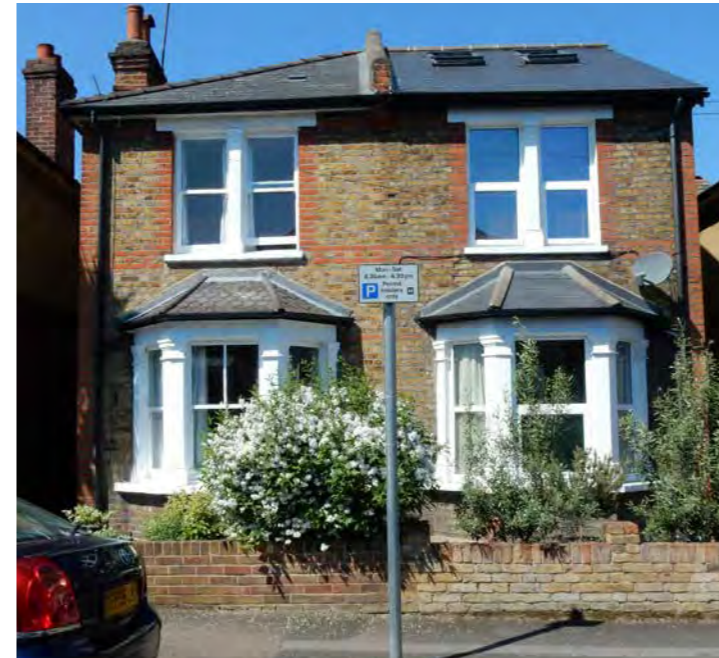
Figure 14: Example of paired windows on Piper Road
