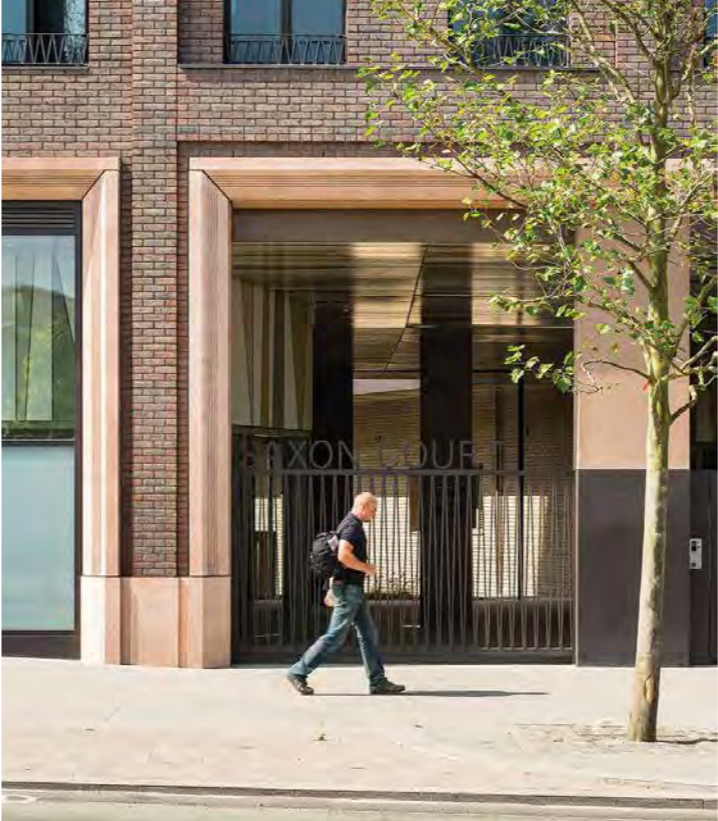
Figure 114: Fenced external lobby, Maccreanor Lavington, Kings Cross November 2020
