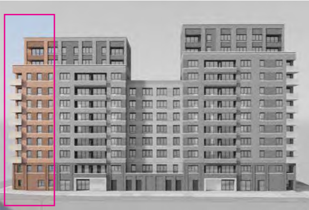
Figure 84: East façades of Buildings E2 and E3
