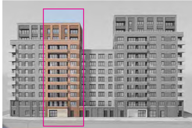
Figure 86: East façades of Buildings E2 and E3
