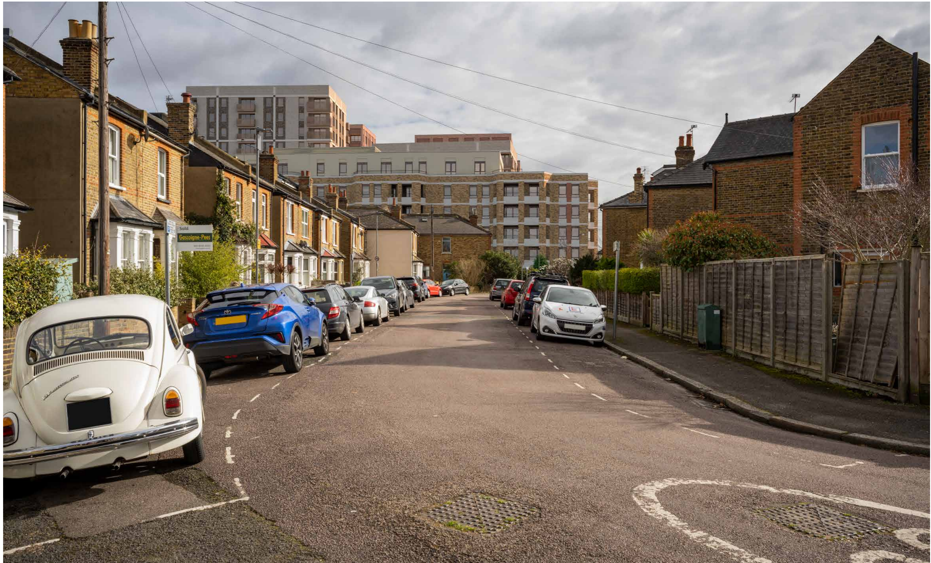
Figure 47: View of Building B within its wider setting. View looking east down Rowlls Road
