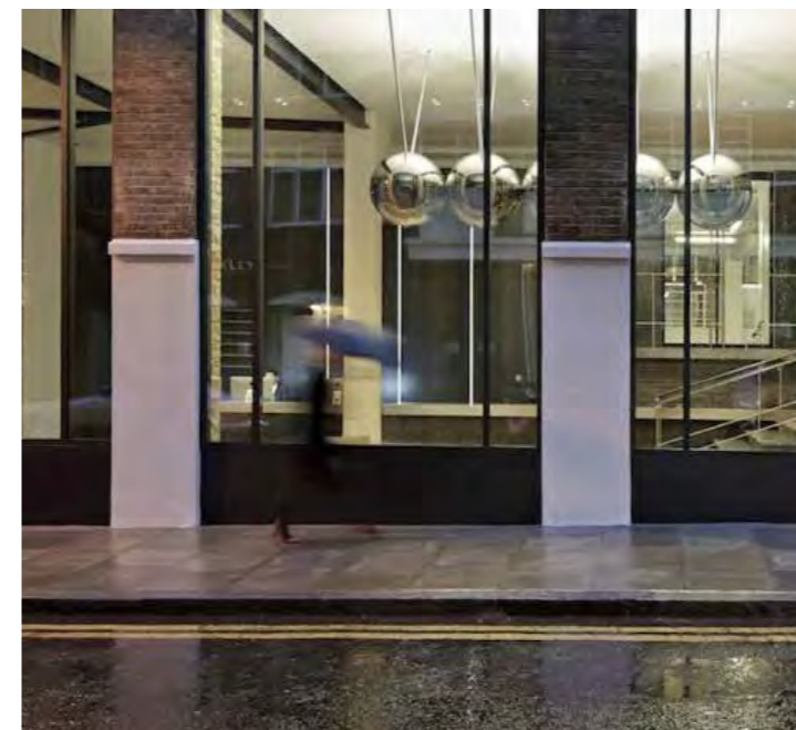
Figure 102: The Buckley Building, Buckley Gray Yeoman November 2020
