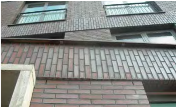
Figure 28: Precedent: soldier and stretcher brickwork
