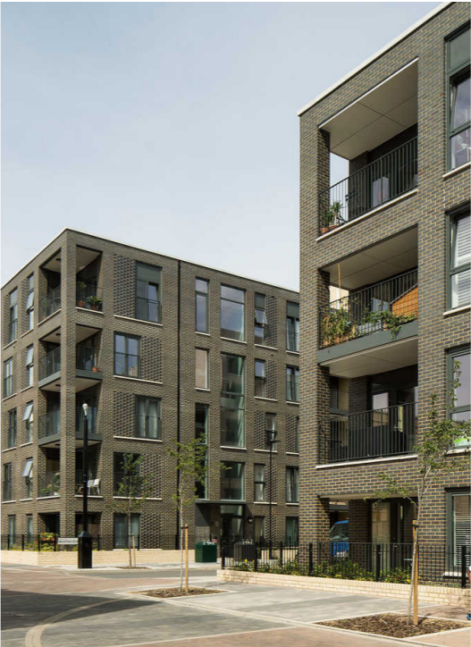
Figure 4.207: Recessed balconies which relate across a street or around an intersection.
