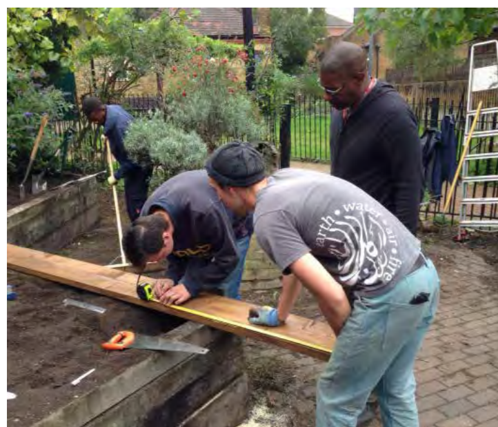
Figure 16: Community construction. Time and Talents, Rotherhithe.
