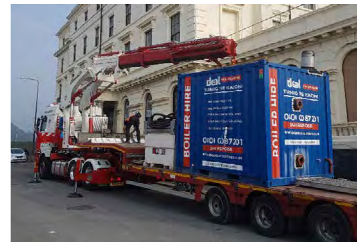
Figure 12: Containerised boiler plant hire.
