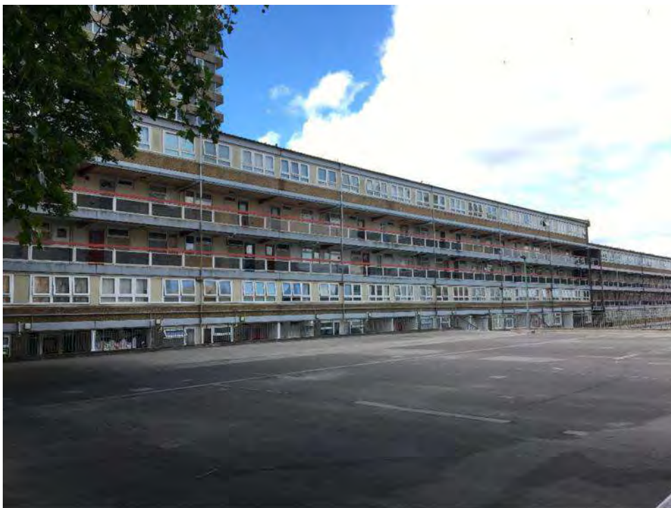
Figure 5.2 Unvegetated areas of hardstanding
